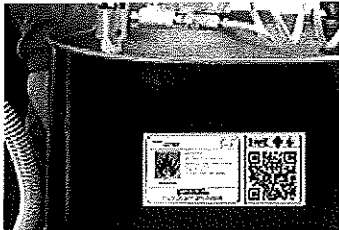
URL encoded QR code linking to Material Safety Data Sheet for hazchems.
